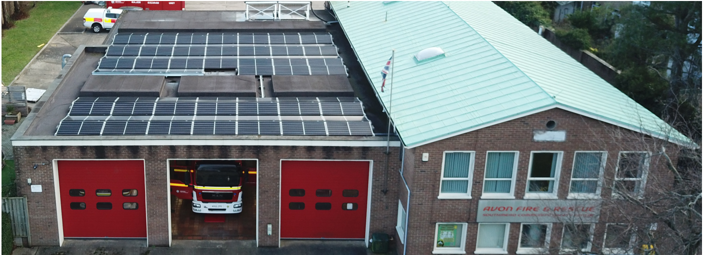
Avon Fire and Rescue Service Clean Energy Project combining solar PV, solar thermal, heat pumps, battery storage and EV charge points.
