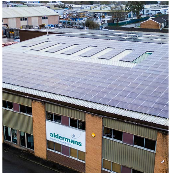
A 263kWp solar PV system installed at Alderman Tooling in Plymouth (estimated to pay back installation costs within 3 years and generate a net profit of £3 million over the next 25 years).
